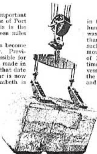
(Top) Concrete block held in position by Fidler's Gear. (Bottom) Meccano model of Fidler's Gear, which reproduces all the movements of the original
